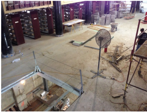
1st Floor has been rebuilt
